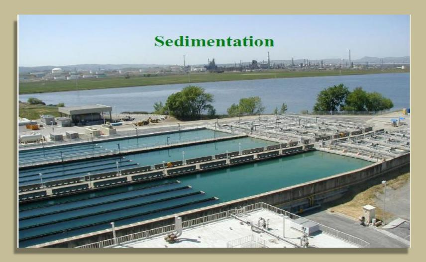
Sedimentation basins are generally made of reinforced concrete, and may be rectangular or circular in plan. A plain sedimentation under normal condition may remove as much as 70 % of the suspended impurities present in the water.
